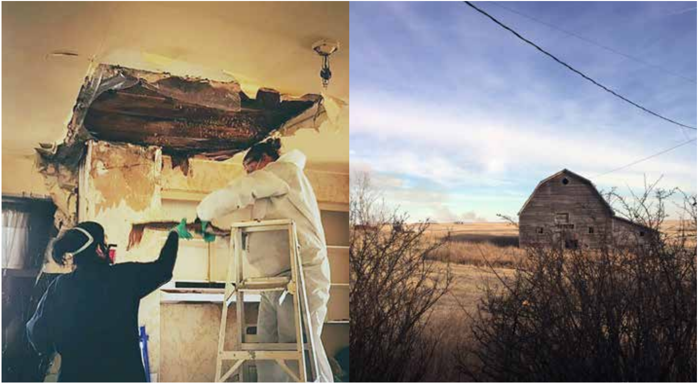
Left: The Haus before/in-progress. Right: view from front porch at The Haus Project
